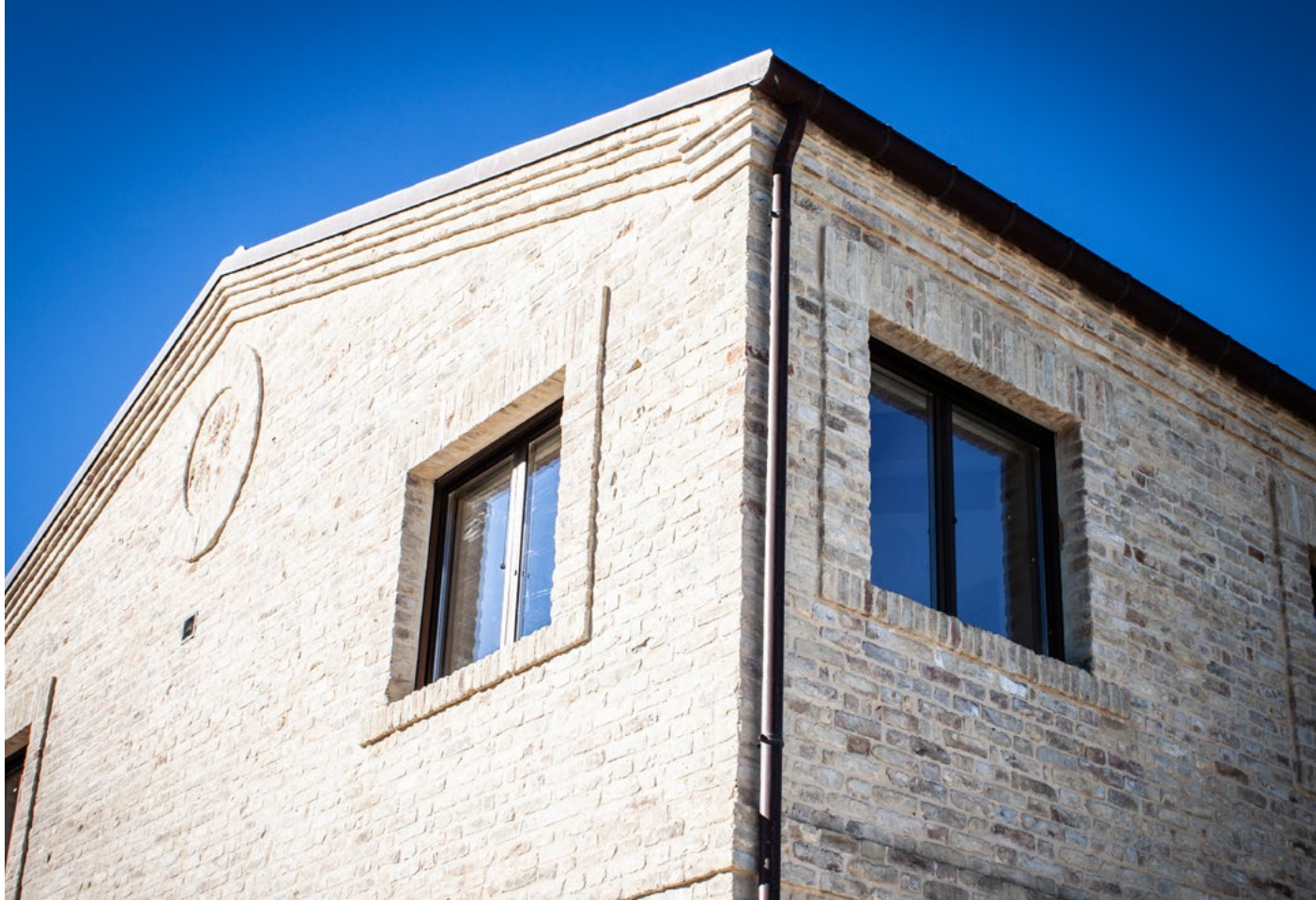
VISTA ESTERNA VILLA PRIVATA IN MOSCIANO, ITALIA Private Villa in Mosciano, Italy
